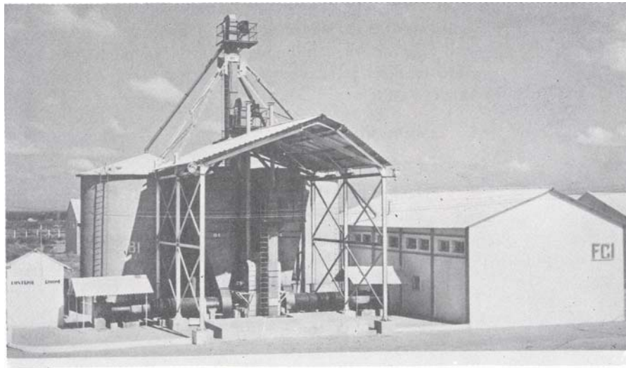
2.25. A commercial drying center using continuous-flow dryers.
