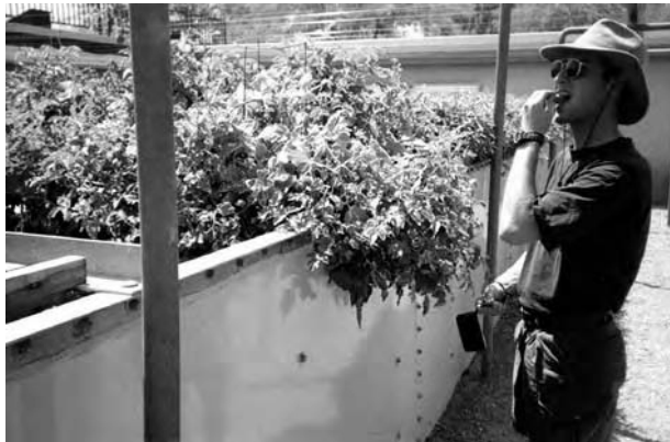
FIGURE 8.2 Tomatoes are being grown in the living machine in Henderson, NV, which treats food wastewater rather than sewage.
