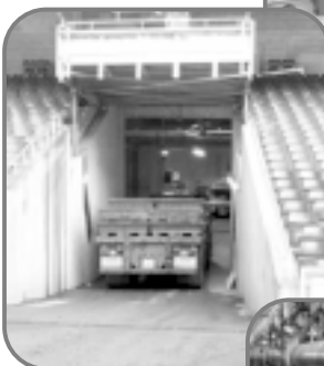
Stadium Access Lift
